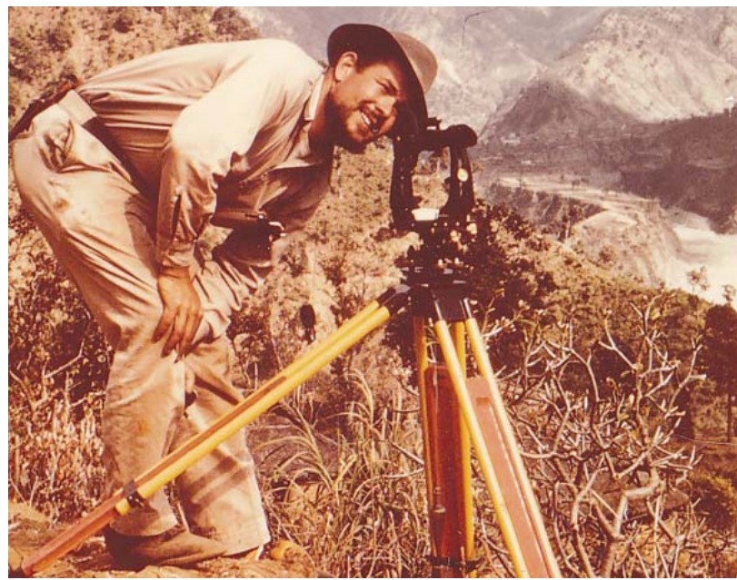
Using a theodolite to survey the route of the ropeway.
