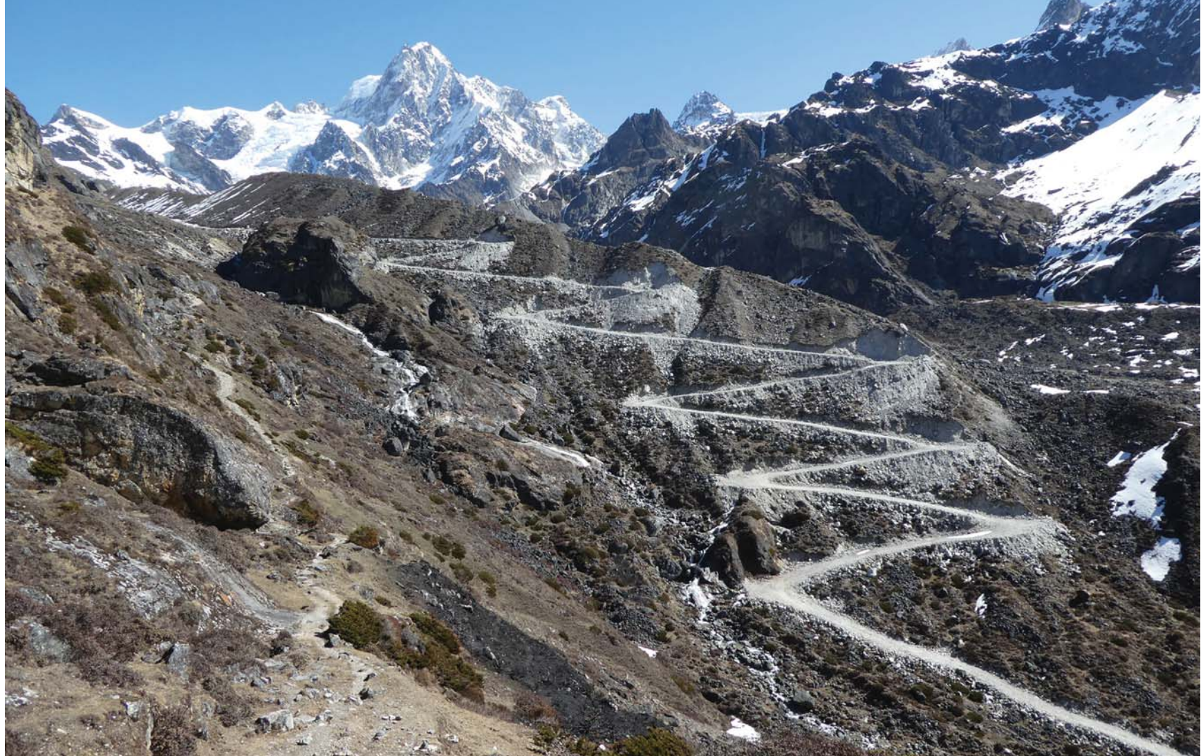
BORDER PASS: Steep switchbacks on a new road from Nepal over the Tiptola Pass up to China.
