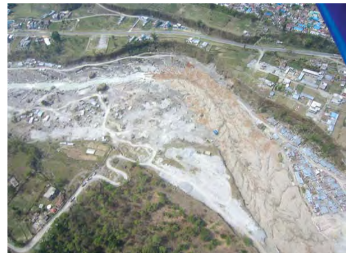
The flood as it raced past the Pokhara-Baglung Highway near Hyangja.
