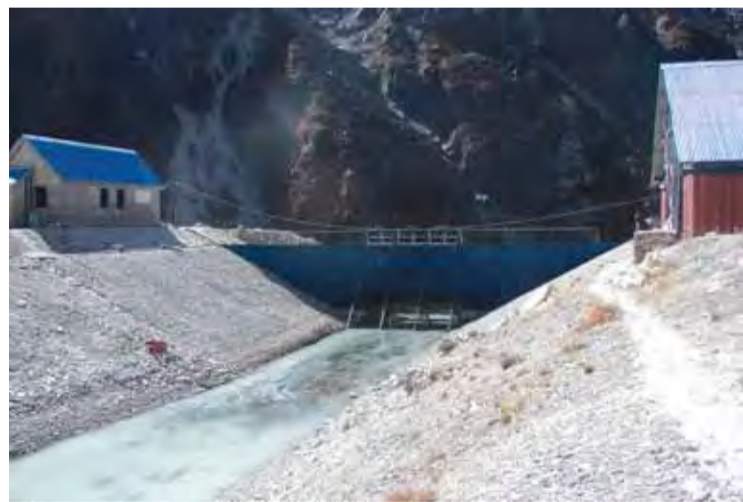
FIRE AND ICE: Global warming melted the ice that made Tso Rolpa so big (top, left), but last week it was frozen solid. Gauri Shankhar towers over the Rolwaling Valley (top) its slopes bereft of snow because of this year's dry winter. The sluice gate of a dam that was built to let out the lake's water to reduce the danger of a catastrophic burst (above).
