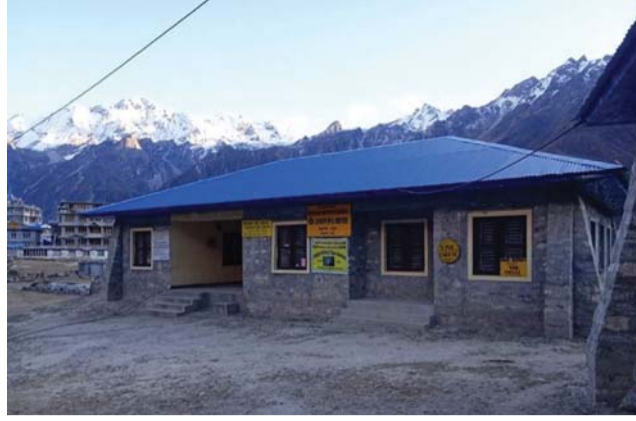
SAY CHEESE: The Kyangjin cheese facility went down in the 2015 earthquake and avalanche. Herders and yaks were killed, all the equipment inside were destroyed. In 2018, the factory was back in operation, with better machinery and a modern lab (left and below).
