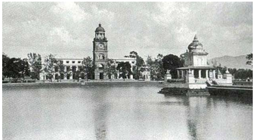
Rani Pokhari and the original Ghanta Ghar clock tower before the 1934 mega-quake that destroyed Kathmandu and killed 10,000 people. Both the clock tower and temple were rebuilt by Jang Bahadur Rana in 1860 in the Moghul dome style.
