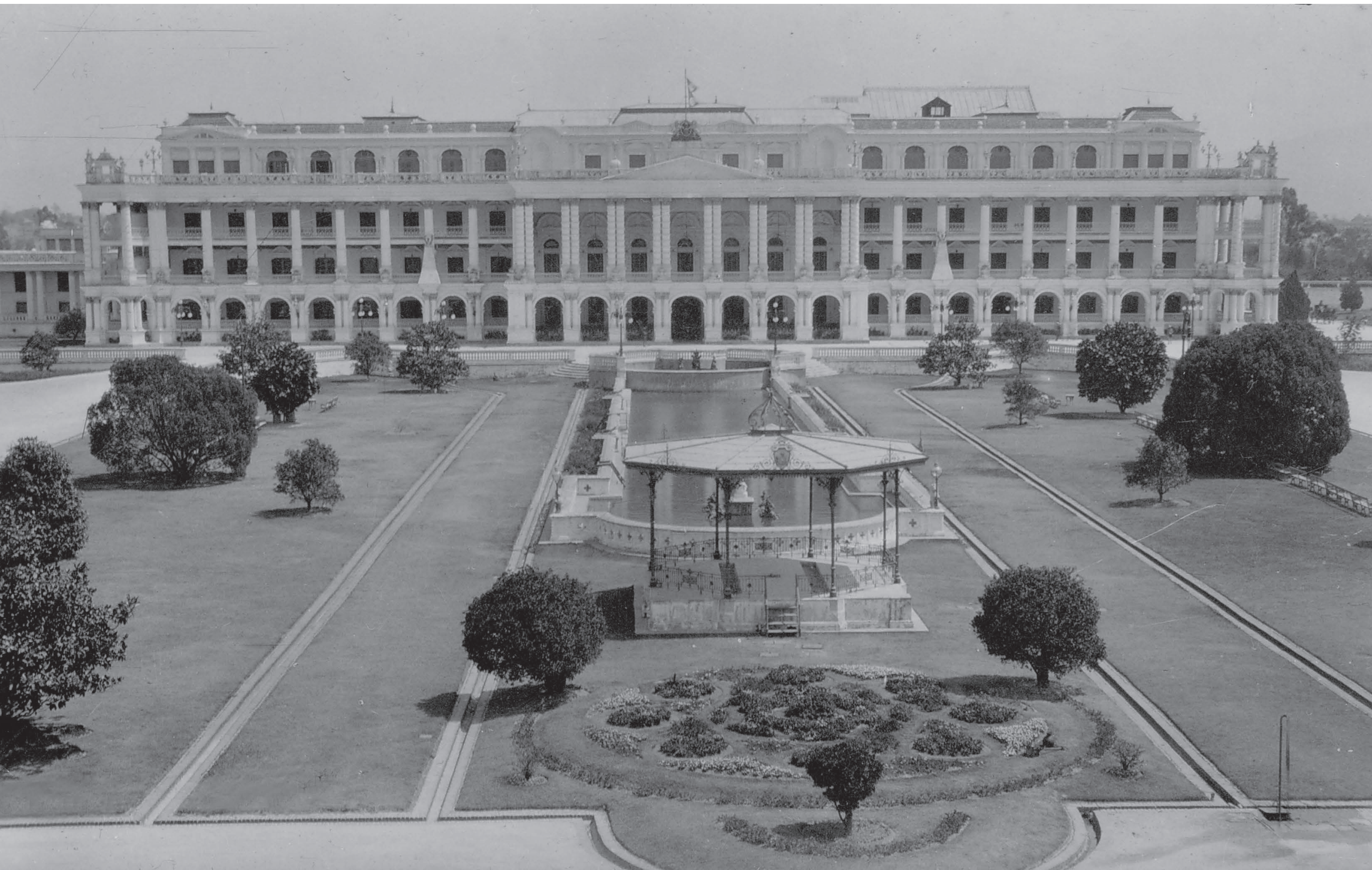
Singha Durbar was built by Prime Minister Chandra Shamsher Rana in 1903, and became the administrative centre of the Nepal government. It was gutted in a fire in 1973 and the main façade suffered structural damage in the 2015 earthquake. MADAN PURASKAR PUSTAKALAYA
