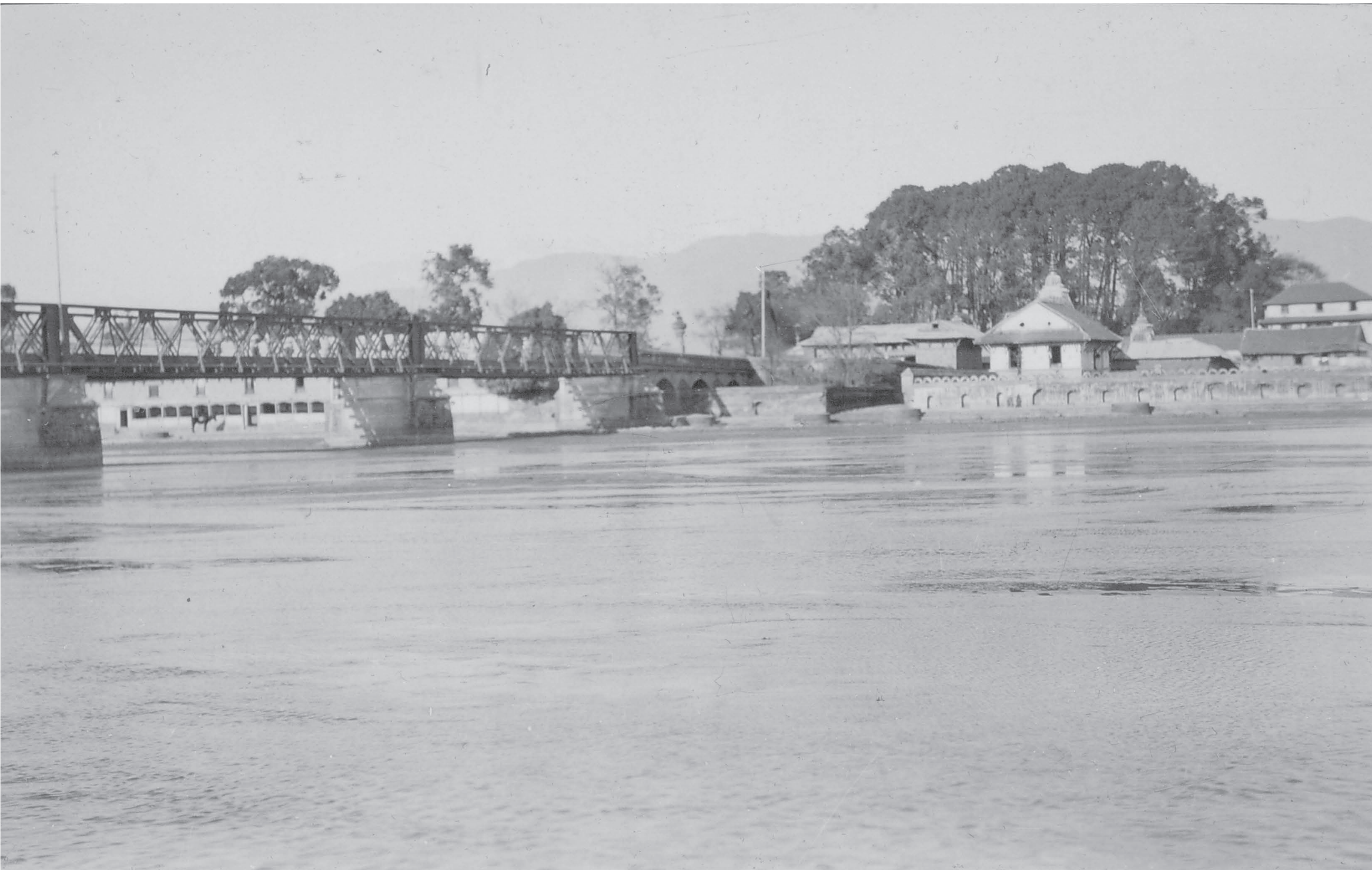
The steel bridge over the Bagmati river as seen from Kopundole in the early 20th century. The bridge was built in England and assembled at the site. MADAN PURASKAR PUSTAKALAYA
